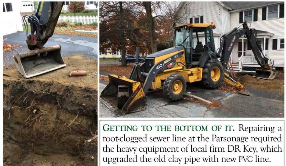
**GETTING TO THE BOTTOM OF IT.** Repairing a root-clogged sewer line at the Parsonage required the heavy equipment of local firm DR Key, which upgraded the old clay pipe with new PVC line.
