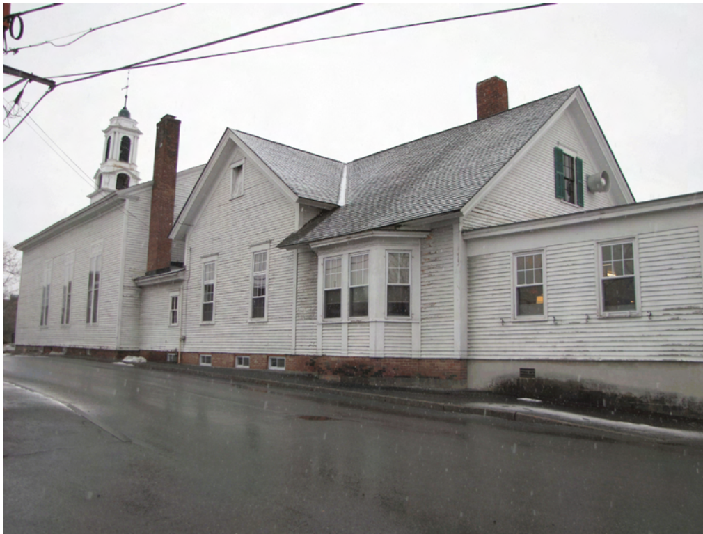
Photo 011: View of west side of building, along street and sidewalk. Note cement parking on 1960's office addition at right side of photo is deteriorated and partially fallen off block.
