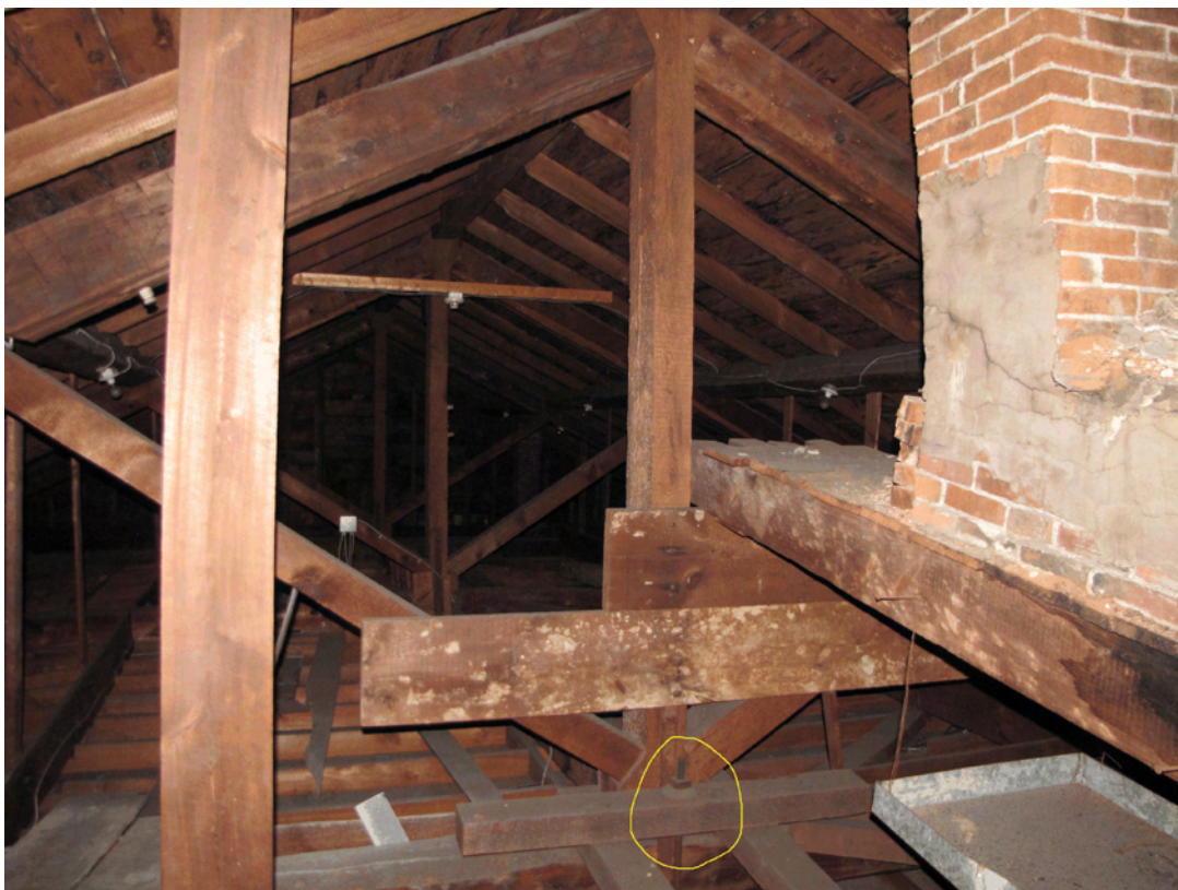
Photo 025A: View showing support of unused brick chimney on truss, plus top of balcony hanger rod in yellow circle.
