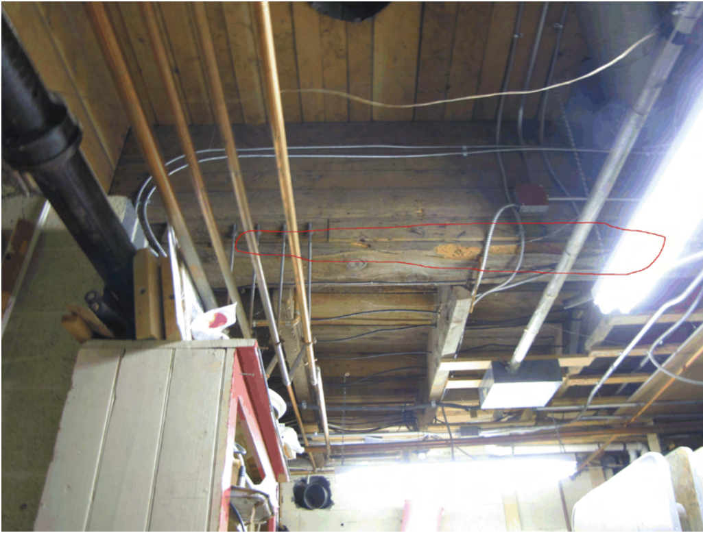
Photo 084A: View of bottom of main floor framing at connector area between sanctuary and fellowship hall showing floor beam with powder post beetle damage in red circled area.
