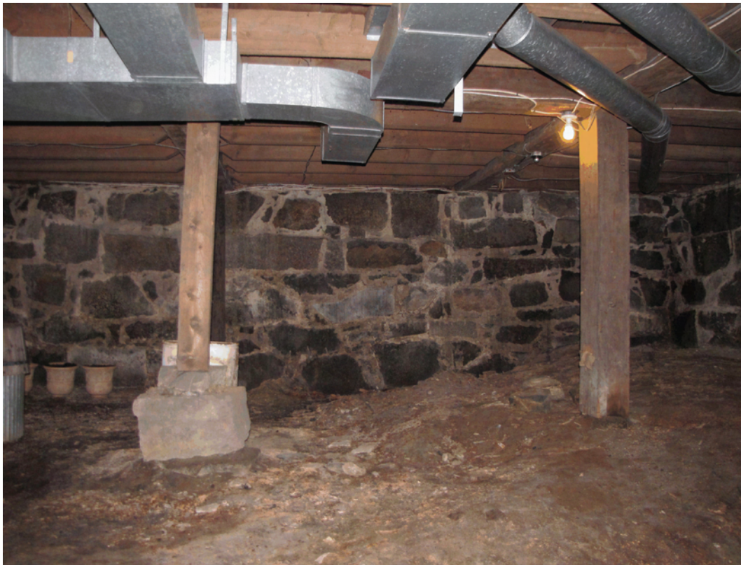
Photo 074: North end of sanctuary basement showing two of four remaining wood posts. Note raised soil grade in right corner. Mortared stone foundation wall appears to be in good condition.
