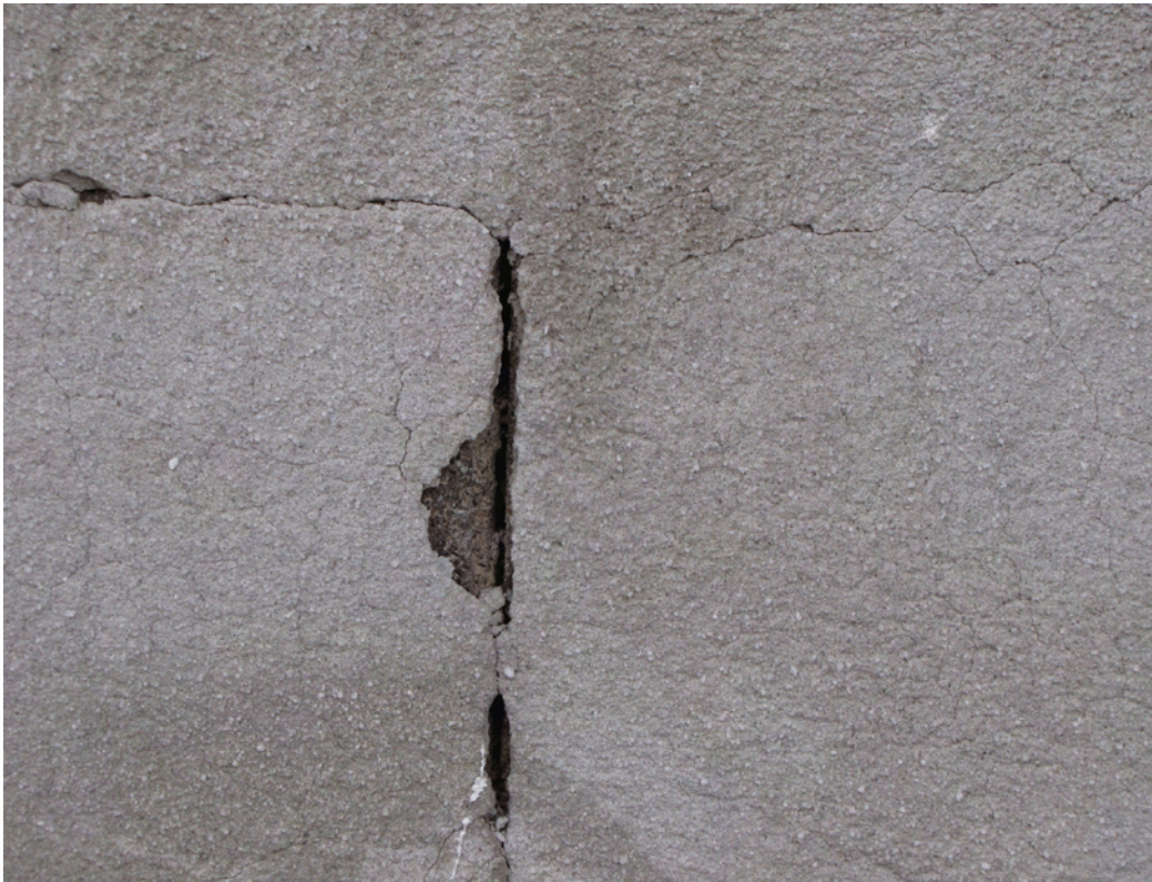
Photo 008: Closeup of 1960's addition deterioration of parging and cracks in masonry block foundation wall.
