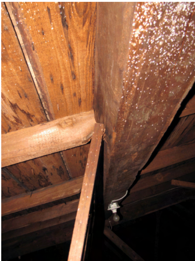
Photo 047A: Attic ceiling and roof framing looking west. Note ceiling joists are notched at diagonal bracing, in yellow circle, which reduces stiffness and increases deflections. Three vertical wood hangers support 1x12 on edge, which supports ceiling joists.
