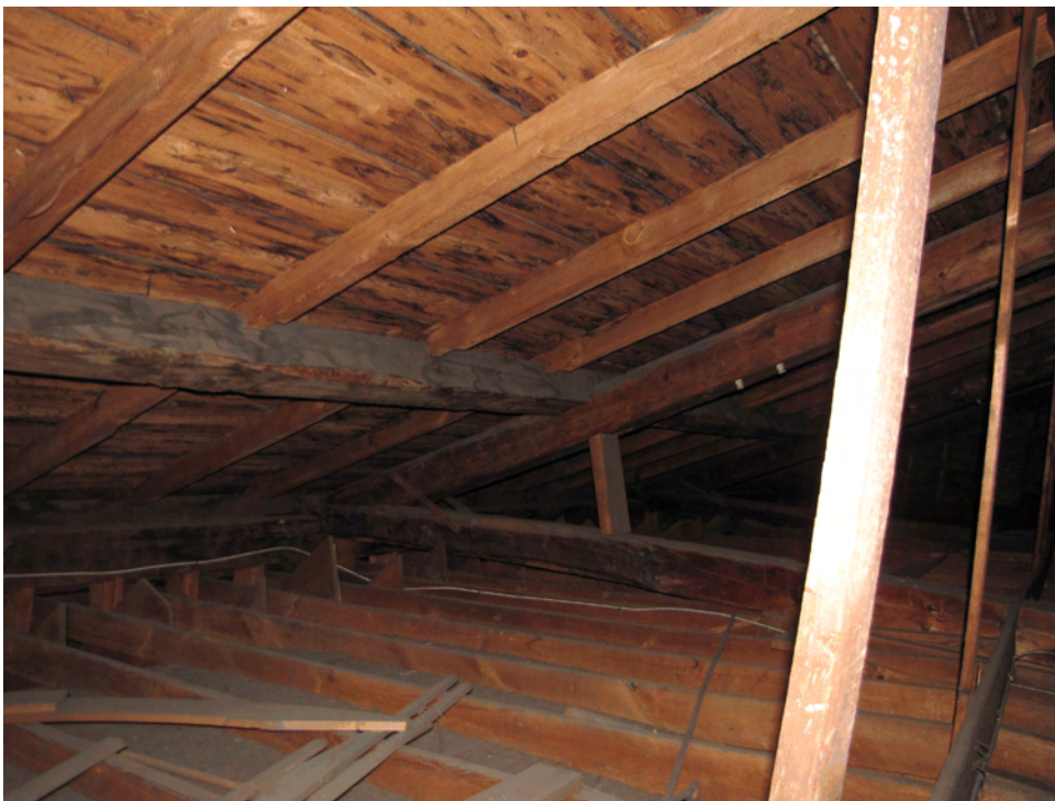
Photo 051: View of east portion of roof, looking south. Note that the ceiling joists have their bottoms cut on a curve, thereby reducing their depth and stiffness near mid-span. Vertical elements on right side of photo are hangers for board supporting the ceiling joists.
