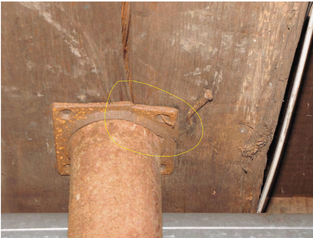
Photo 073A: Closeup view of sanctuary basement lally column support where the cap plate is cracked and displaced. The cap plate should be replaced.
