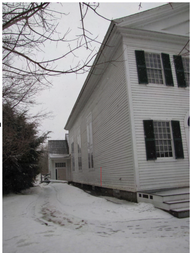
Photo 020A: View of east side of sanctuary portion of building. Note change of foundation wall at red line from granite stone to brick on concrete.
