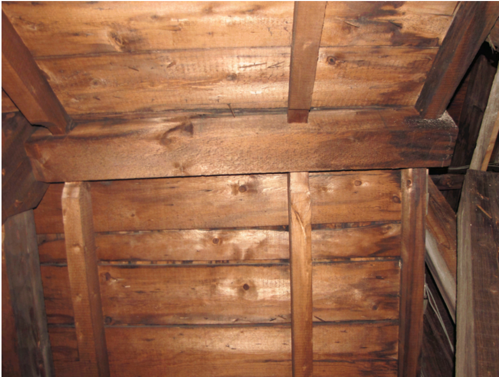
Photo 026: Short ridge beam between 1 st roof truss from north wall and steeple/cupola wall framing. Right end of ridge beam is unsupported.
