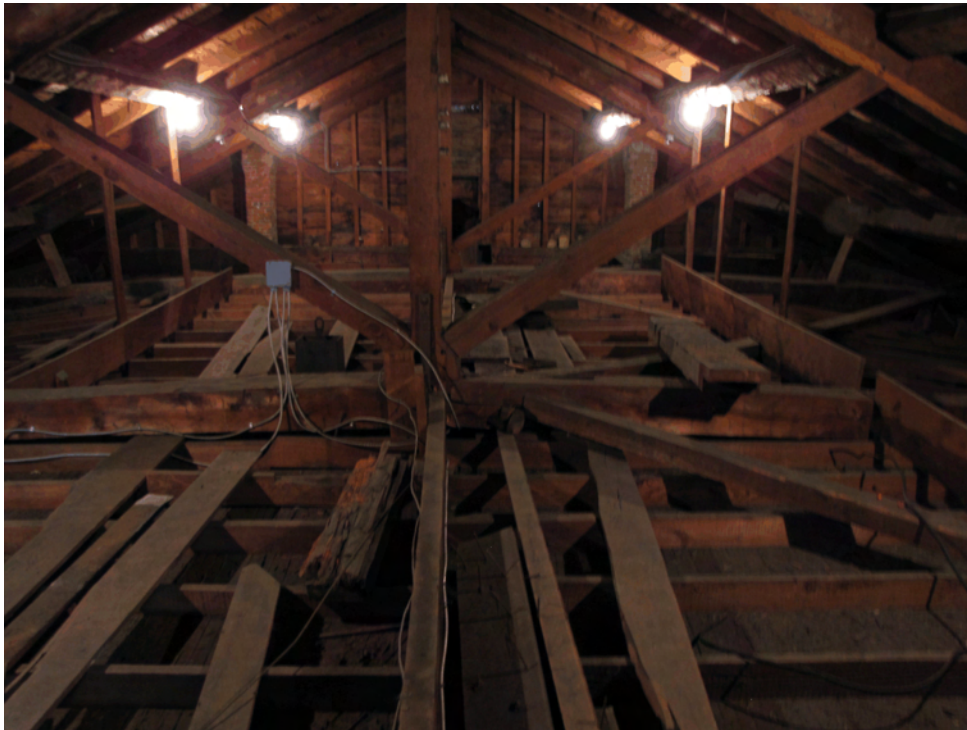
Photo 054: Interior view of sanctuary roof framing looking south. Heavy timber roof trusses clear span the sanctuary in an east-west direction. Note the ceiling joist framing with lath (for plaster) directly attached and no insulation.
