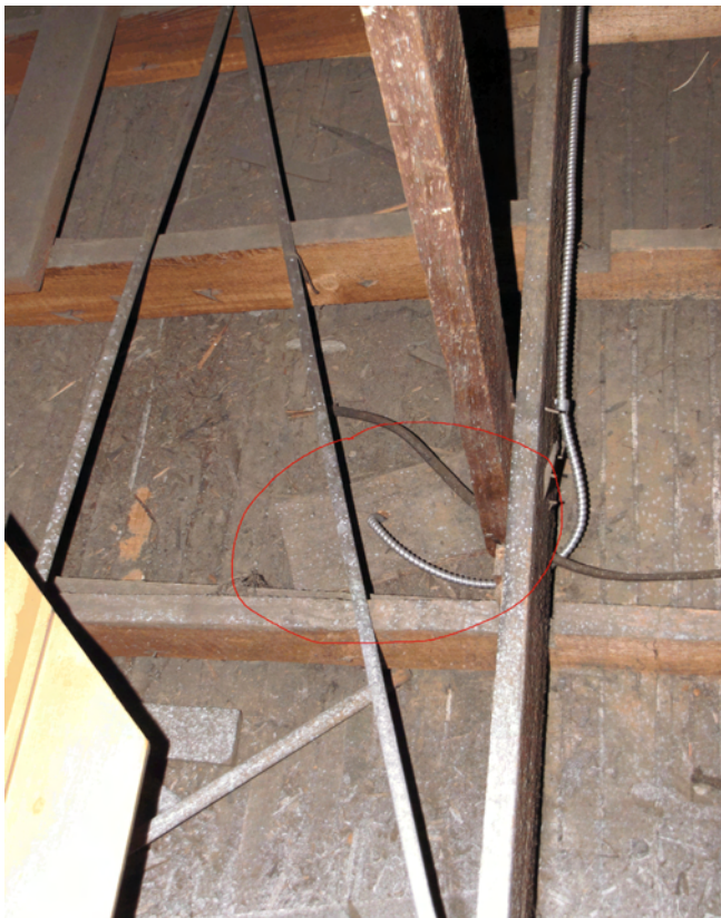
Photo 059A: Attic ceiling framing with electric wire at center in red circle feeding hung chandelier in sanctuary. Note that added wood plate from which the chandelier is supported, is in turn only supported by the wood lath, not the ceiling joist framing.
