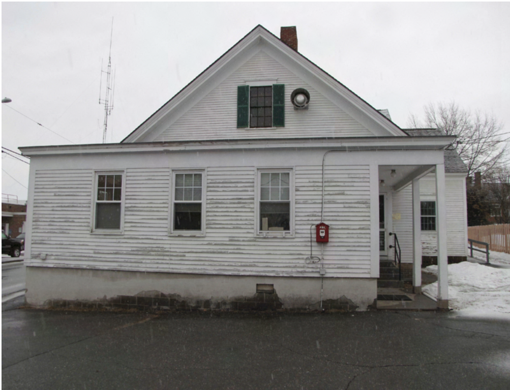
Photo 009: View of south end of the building, at the 1960's addition. Note cement parking has partially cracked and fallen off the masonry block foundation.
