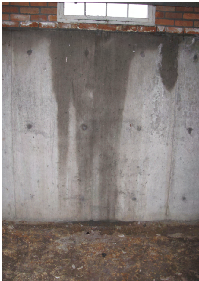
Photo 080: West wall of sanctuary basement showing dampness on wall from water infiltration at bottom of brick.
