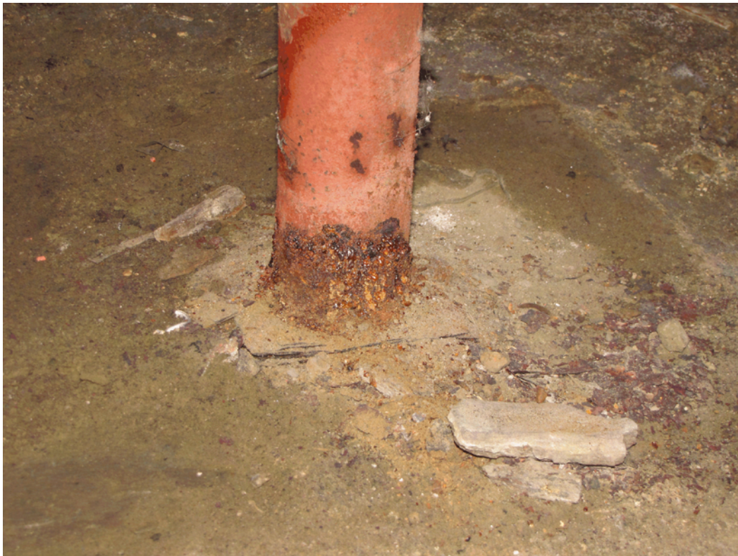
Photo 078: Closeup view of sanctuary basement lally column base with corrosion.
