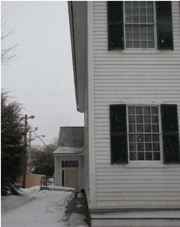
Photo 022: Looking south along east wall of sanctuary with vertical bow in wall visible, which results from diagonal ceiling framing horizontal load component.
