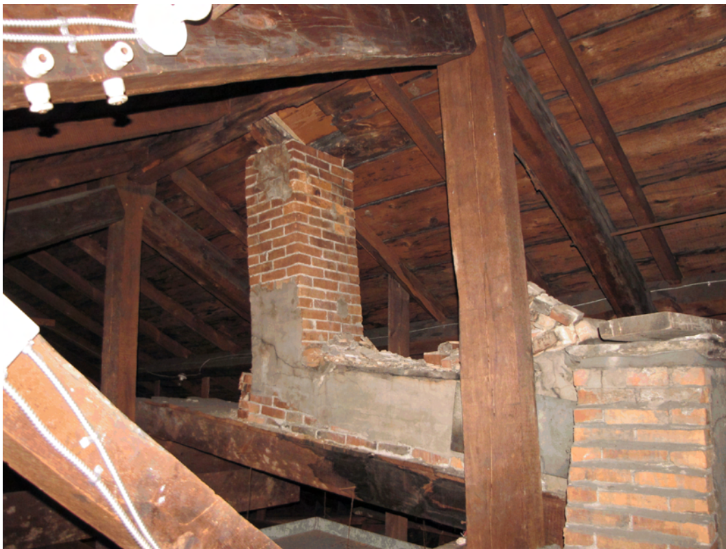
Photo 024: Old unused brick chimney should be removed to reduce weight on structure.
