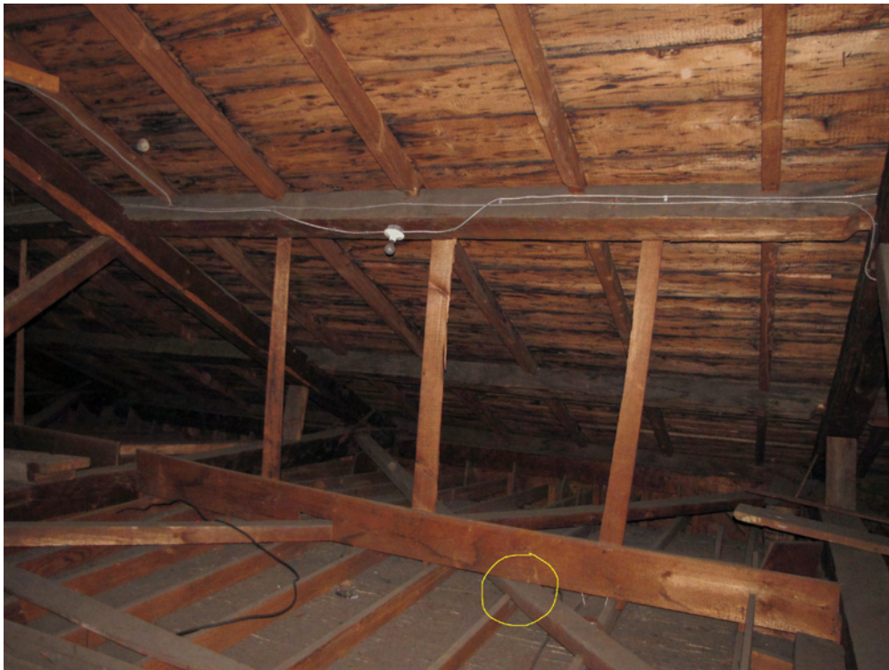
Photo 047A: Attic ceiling and roof framing looking west. Note ceiling joists are notched at diagonal bracing, in yellow circle, which reduces stiffness and increases deflections. Three vertical wood hangers support 1x12 on edge, which supports ceiling joists.
