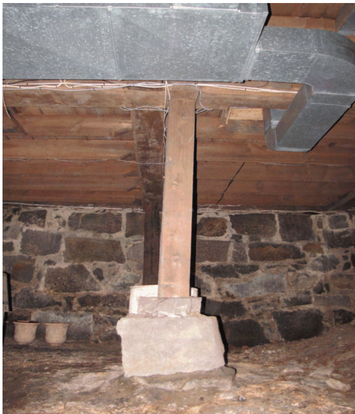
Photo 074: North end of sanctuary basement showing two of four remaining wood posts. Note raised soil grade in right corner. Mortared stone foundation wall appears to be in good condition.
