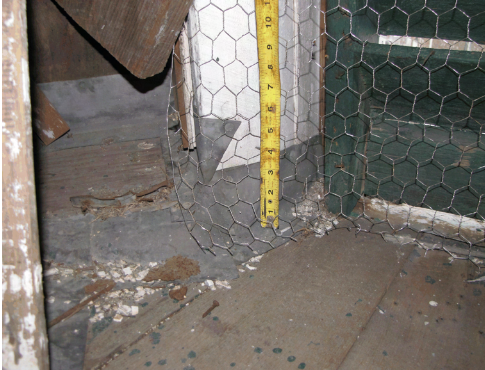
Photo 032: Flashing around corner posts at walls below upper cupola. Note flashing extends down to wood roof boards. There is no waterproof membrane on this partially protected roof.
