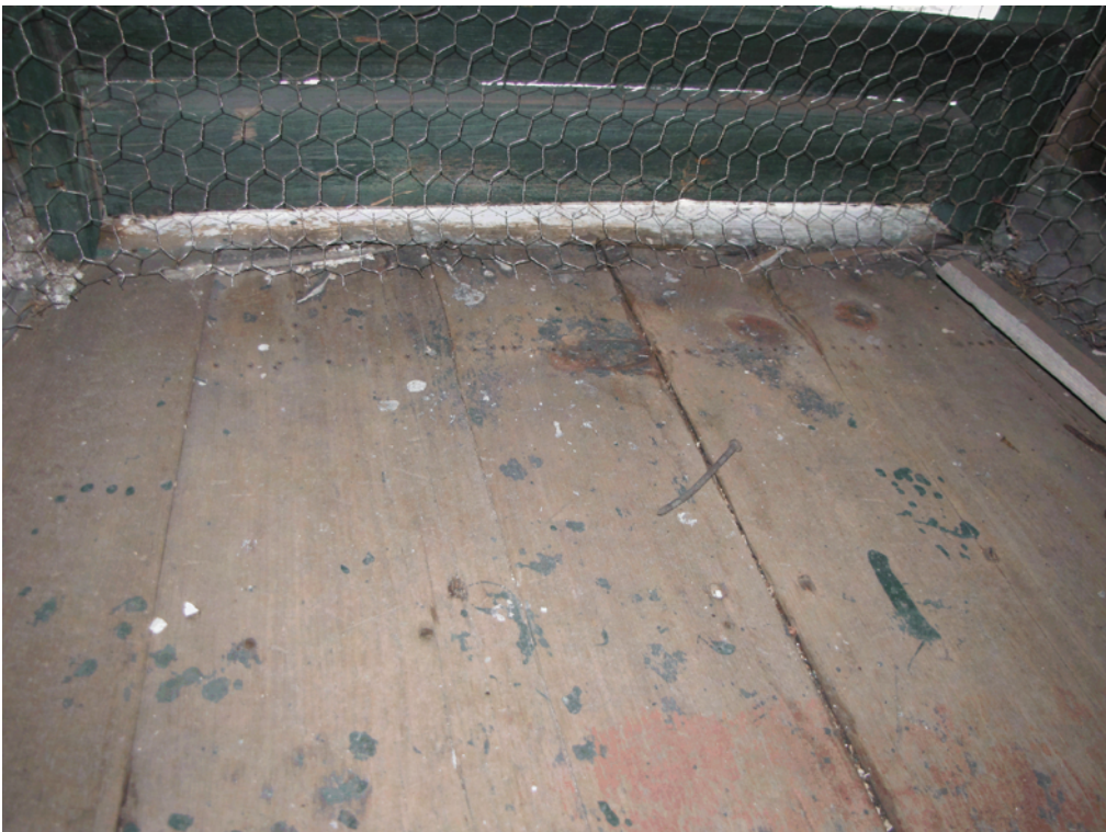
Photo 031: Roof over bell showing exposed wood plank roof which is highly susceptible to wind blown rain/moisture.
