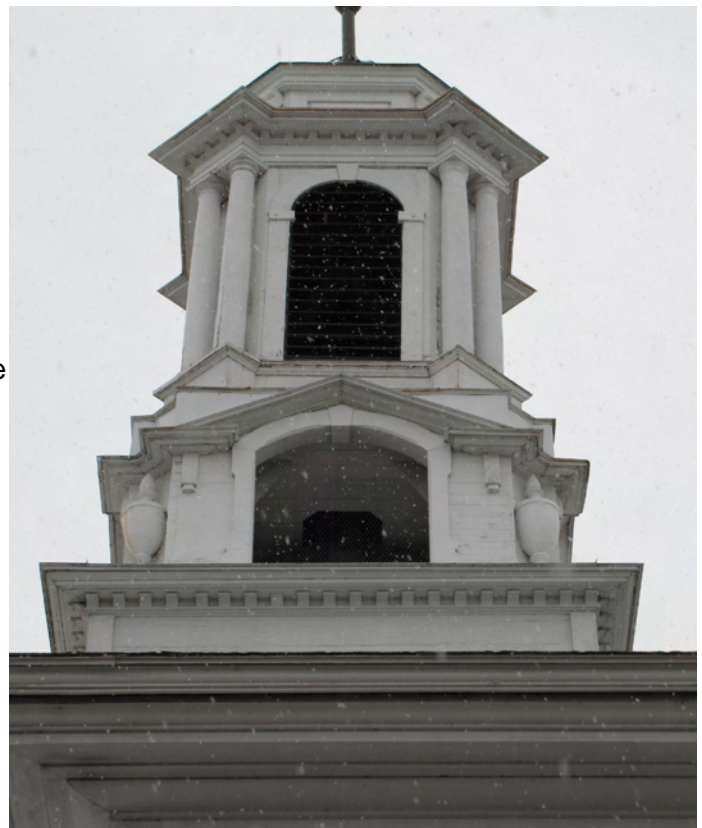
Photo 014: Steeple and cupola, viewed from the west, showing slight tilt towards the rear of the building, as a result of interior beam support deflections.
