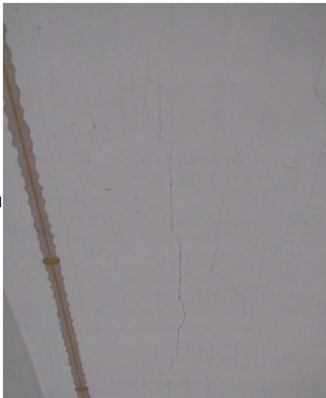
Photo 061: Sanctuary ceiling plaster cracks running north-south, which occur at both east and west sides of the sanctuary.
