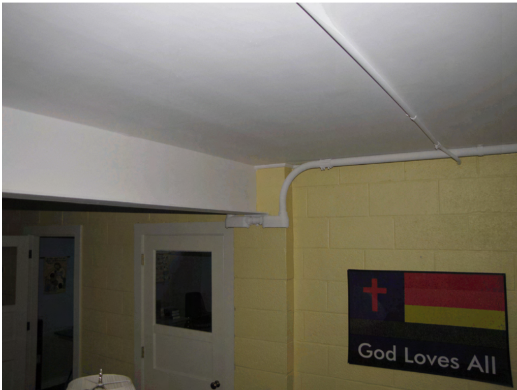
Photo 085: Lower level of 1920's addition showing a portion of the steel floor beam projecting below the ceiling. Hump visible at the top side of the floor, occurs at this floor beam.
