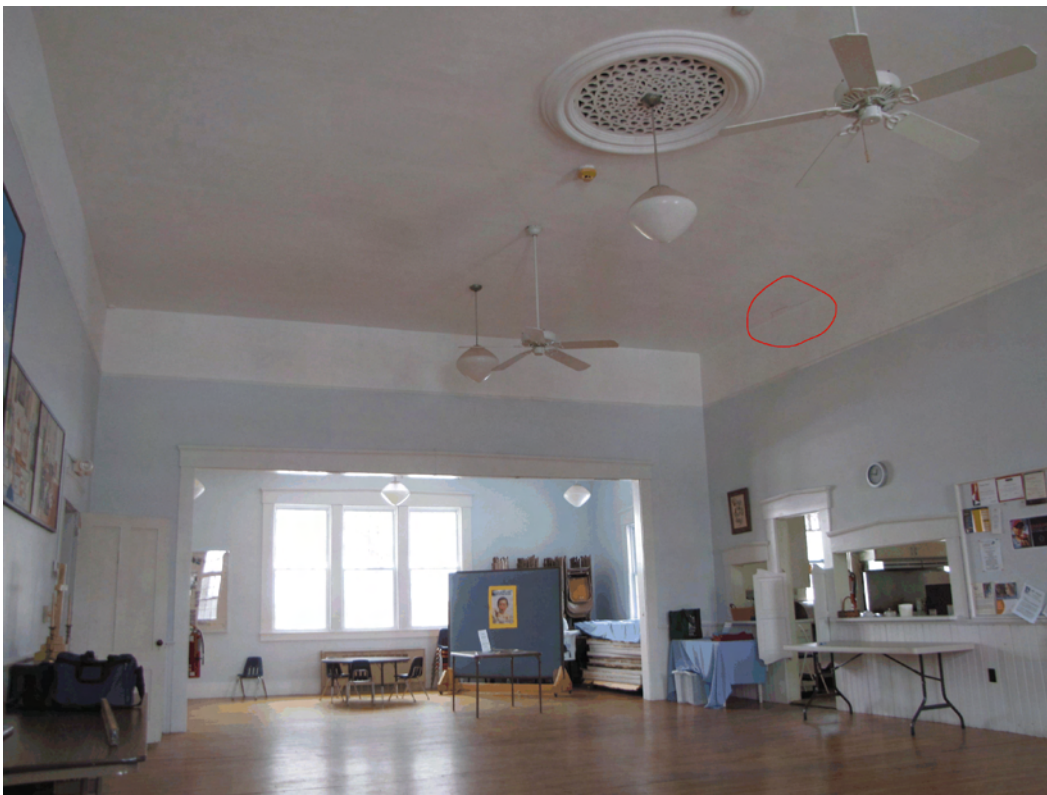
Photo 092A: Interior view of 1920's addition looking east. Walls and ceilings are in good condition with sole exception of ceiling cracks in red circled area.
