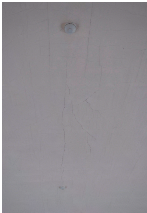
Photo 060: Sanctuary ceiling plaster cracks between and around smoke detectors.
