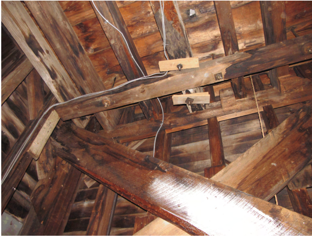
Photo 035: Under side of bell floor framing at steeple/cupola, showing tension rods in wall to resist structure overturning and rod bottoms in upper half of photo which tie the upper cupola framing down. Note wood framing appears to be in good condition.
