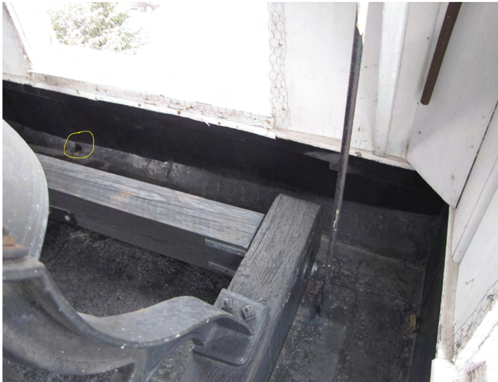
Photo 033A: Floor of bell area. Note drain hole for water in yellow circle, located at the south wall of the steeple, is at the high point of the sloped framing, reducing the effectiveness of the drain.
