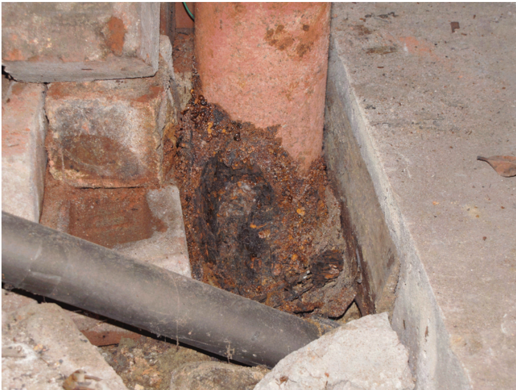
Photo 079: Closeup view of lally column base by furnaces with severe corrosion and material loss - steel jacket and some inner concrete.
