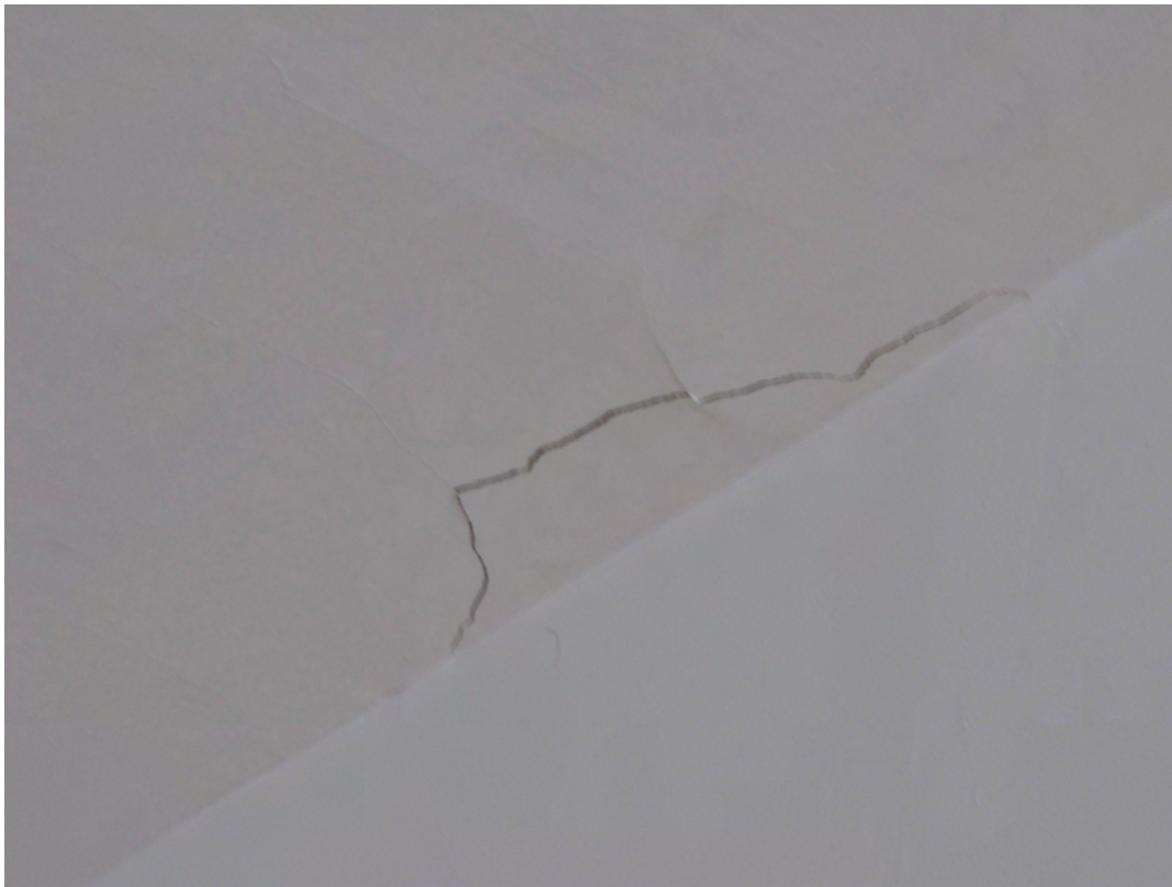
Photo 091: Closeup view of cracked plaster ceiling from Photo 092A.
