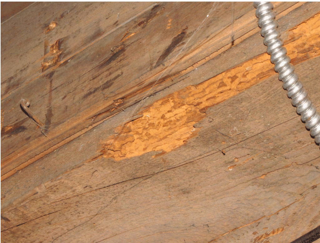
Photo 083: Closeup of damage to wood floor beam by beetle infestation.
