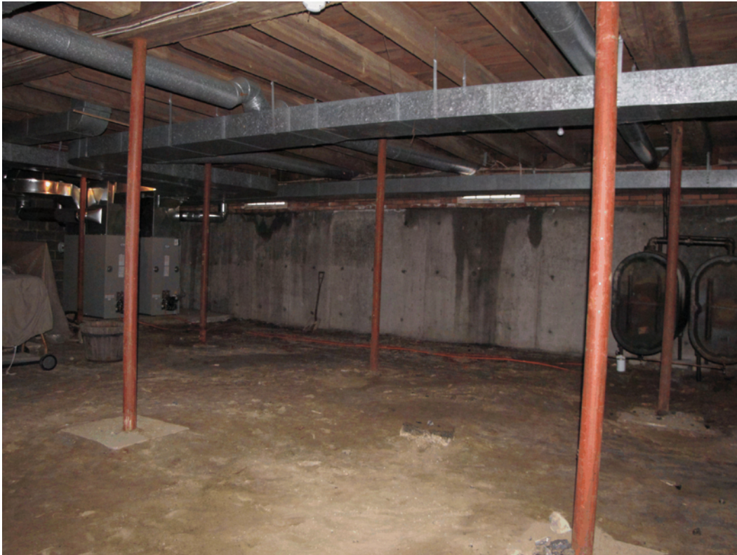
Photo 071: View of basement area beneath sanctuary, looking southwest. Note small size of footings which are flush with the soil grade.
