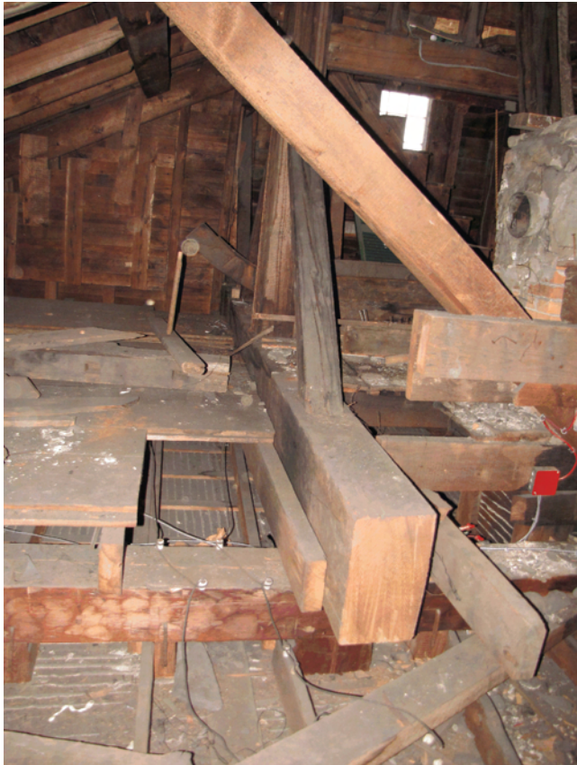
Photo 099: View looking north in attic, showing transfer beam that supports steeple/cupola framing bearing on bottom chord of roof truss (running right-left near bottom). Note this roof truss has interior post supports beneath it, making deflection differentials between it and the next truss to the south (supporting the balcony) more pronounced and greater. Note lack of any insulation on top of the plaster and lath ceiling.
