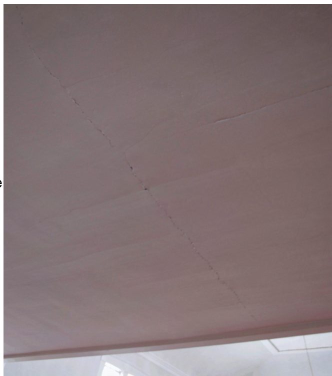
Photo 064: Cracking in plaster ceiling at the underside of the balcony.
